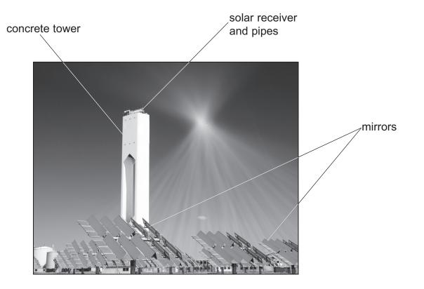
Mirrors are used to direct the Sun's rays onto the solar receiver at the (a) top of the tower.
